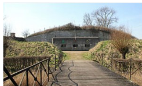
Fort Penserdijk Tinte
